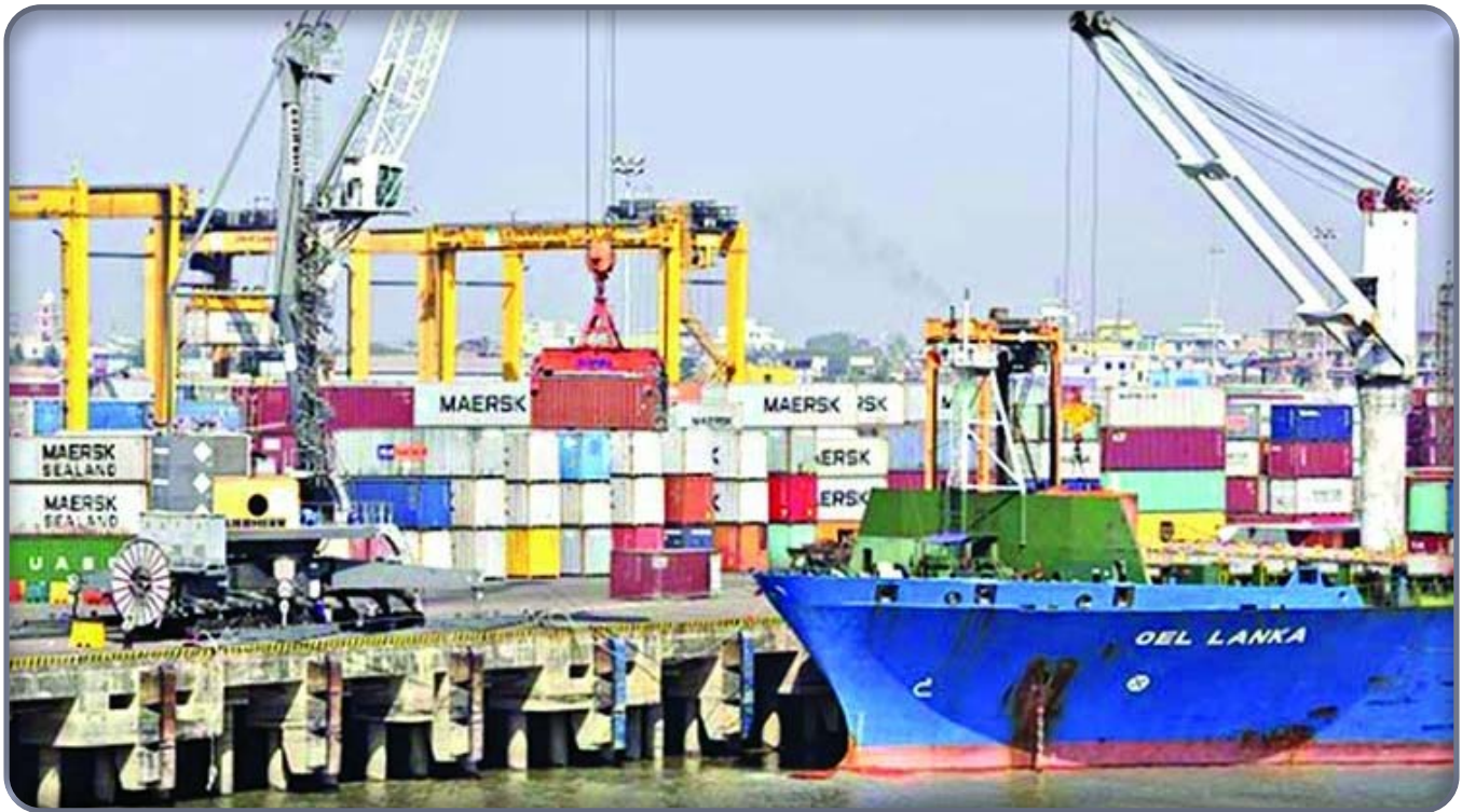
Figure 12: Construction of Matarbari Deep Sea Port
