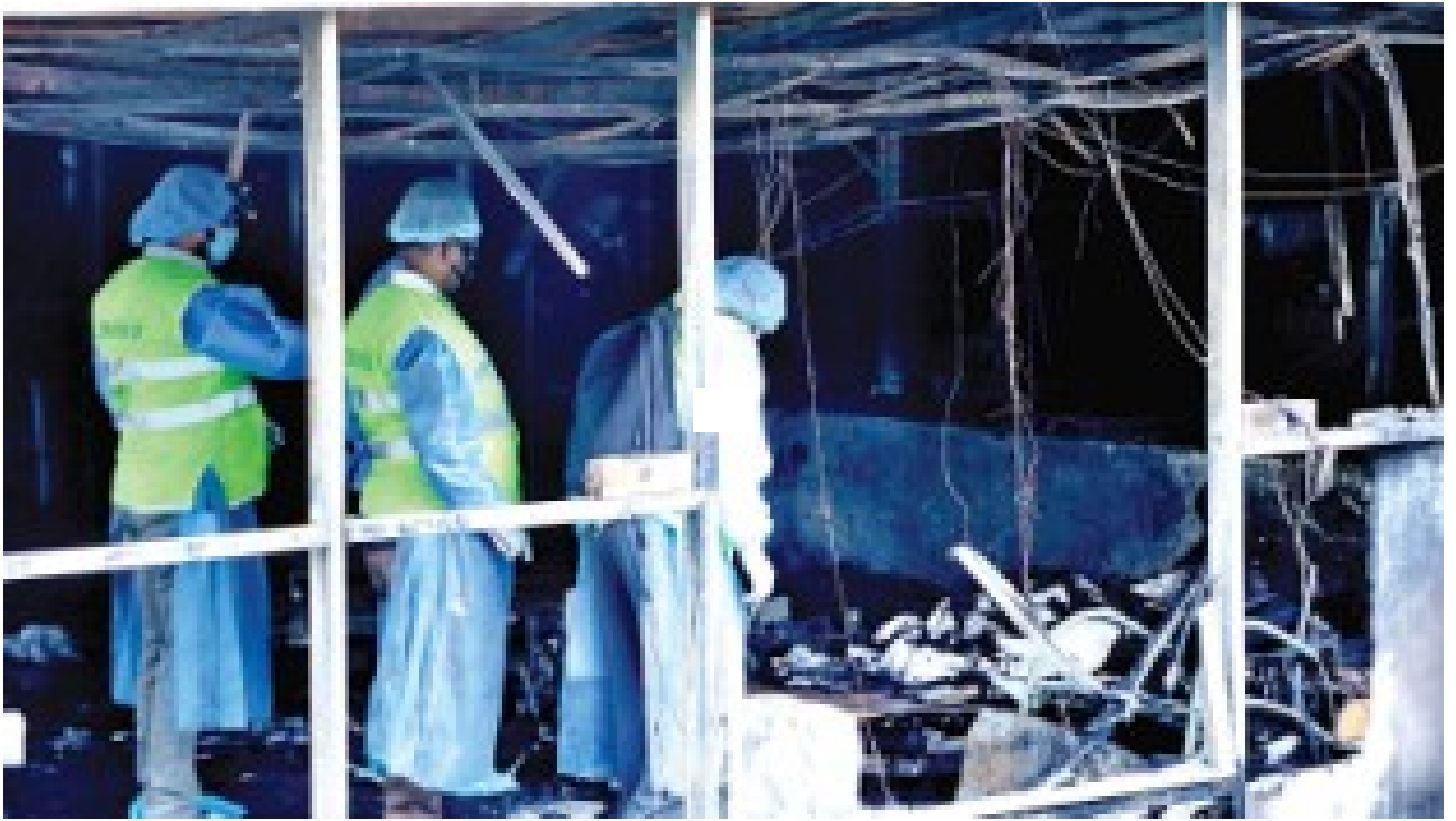
Fatal Blaze at United Hospital: Burnt unit had no fire safety
