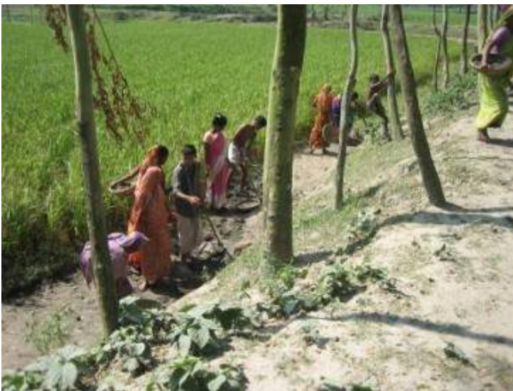
Men and women digging earth
