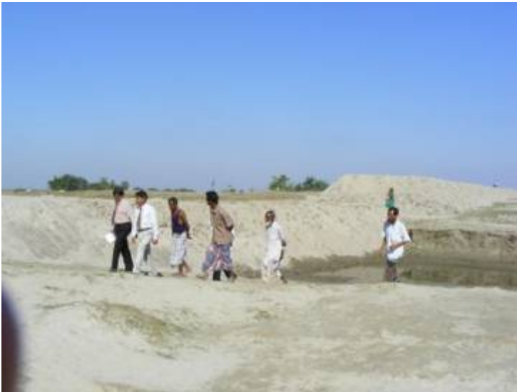
Ministry officials visiting a 100-Day EGP work site
