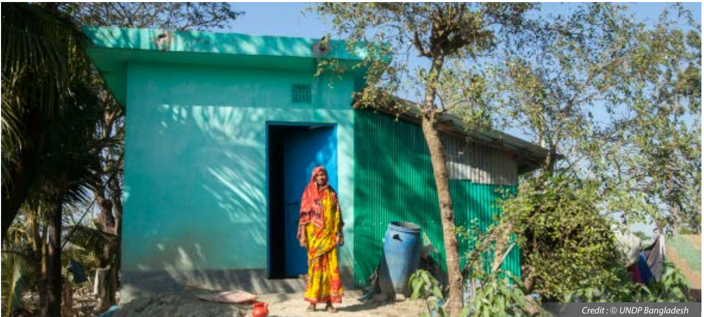
Flood proofing through raising homestead plinth level
