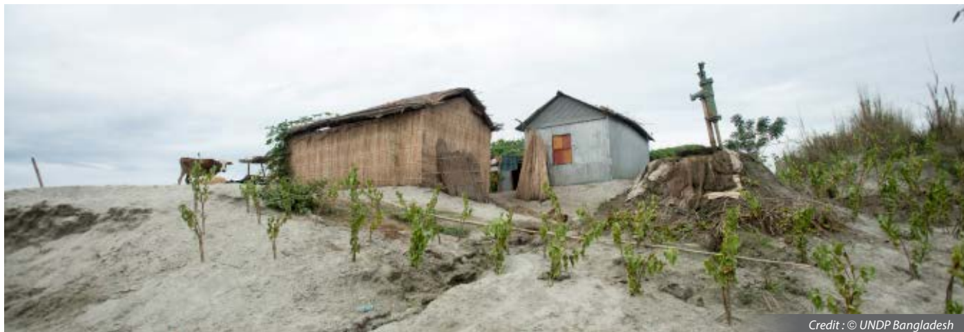
A dilapidated house in the Chars of Kurigram
