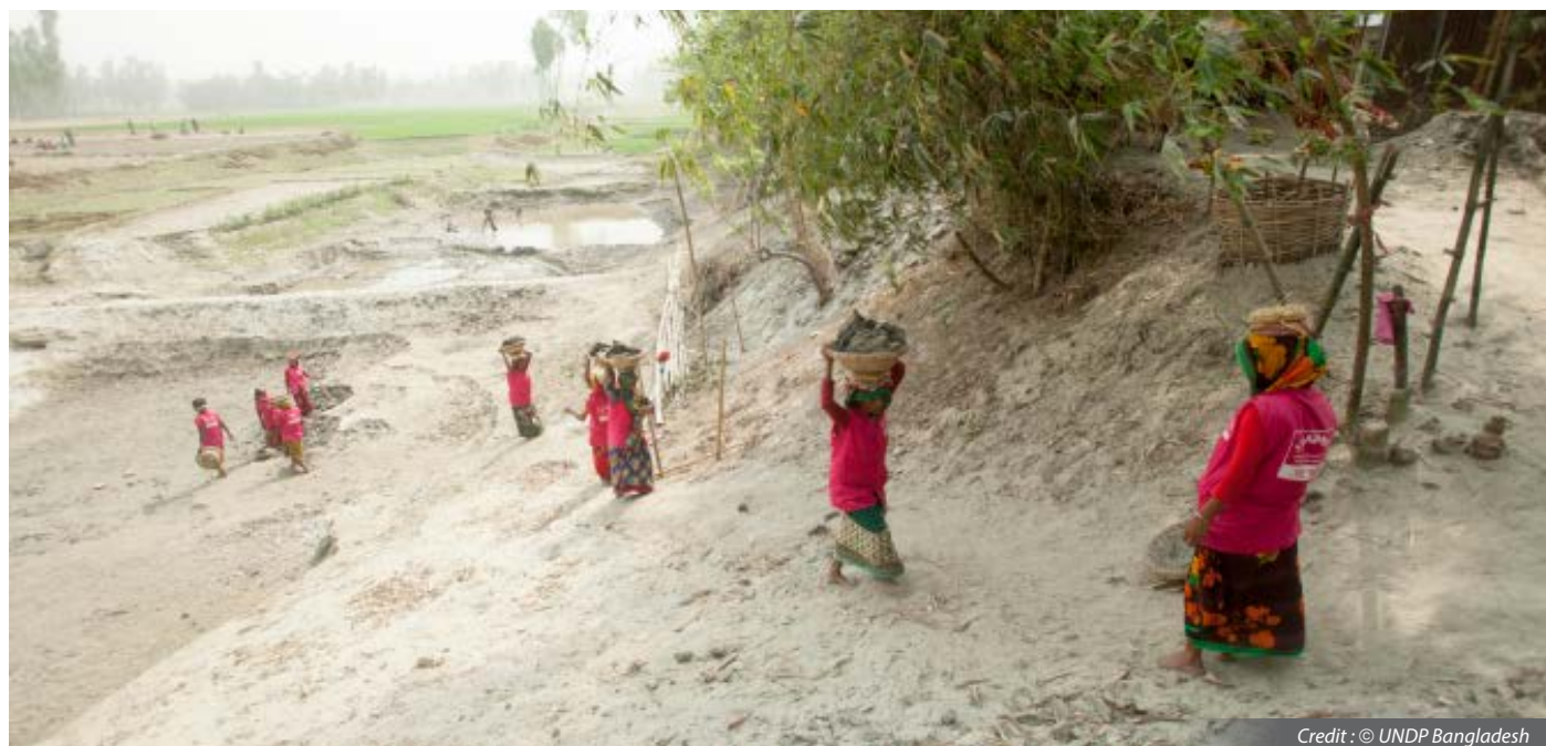
Women engaged in road construction in Kurigram as part of the SP schemes of LGD
